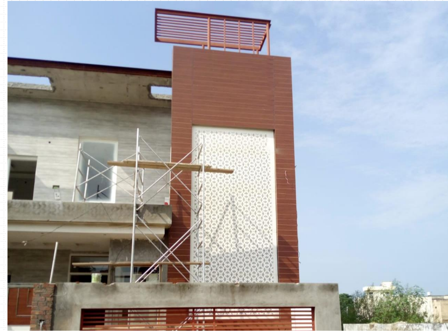
WORK ON PROGRESS
