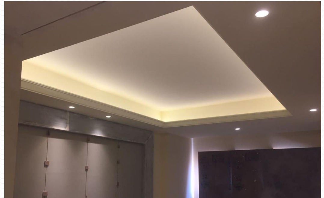
WORK ON PROGRESS
