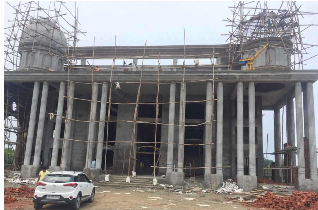
WORK ON PROGRESS
