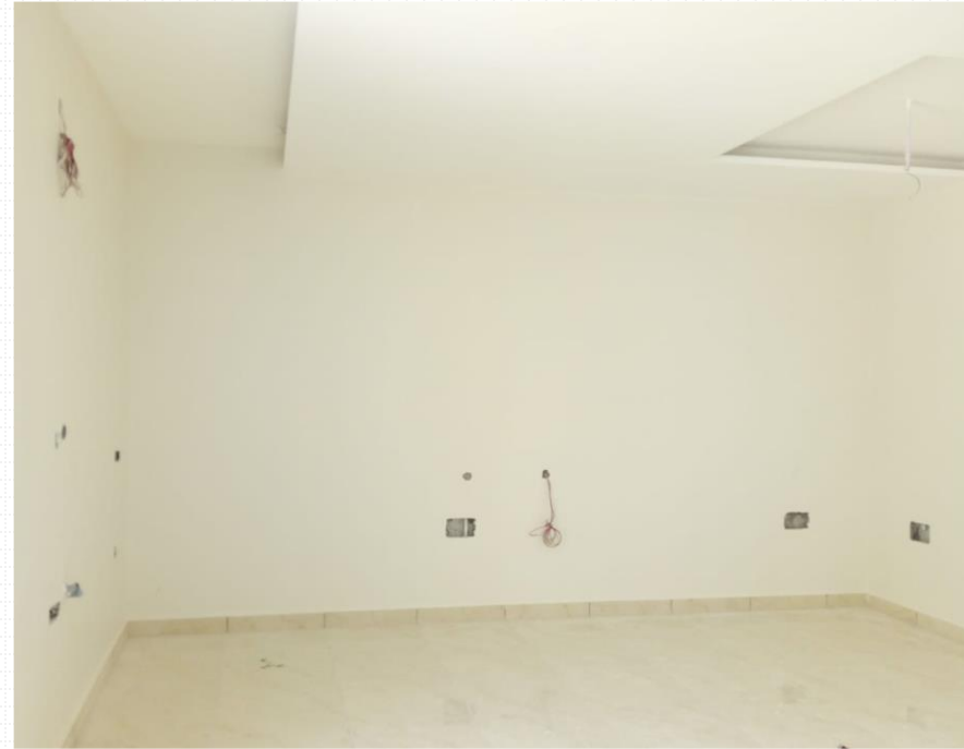
WORK ON PROGRESS
